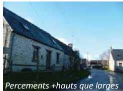
Percements +hauts que larges
